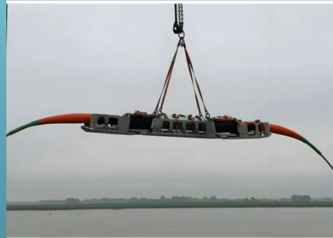
Submarine joint closure
